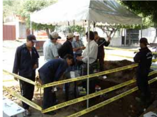
Photo-4 Flow Meter Installation Arrangement where Inlet Pipe was dug out
