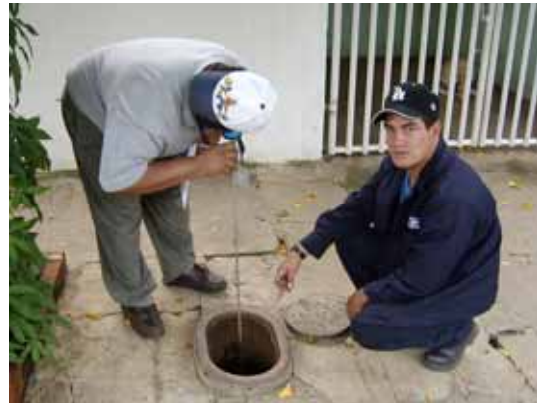
Photo-8 Sound Listening Check of Service Line
