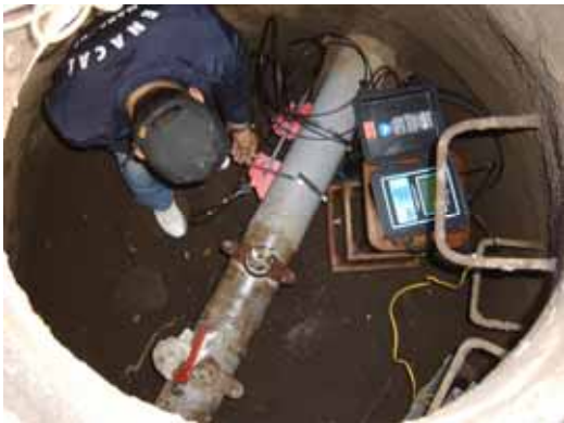
Photo-3 Flow Meter Installation on Inlet Pipe Manhole is available
