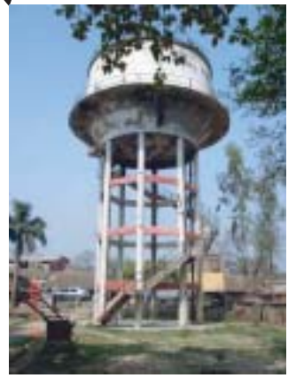
Existing elevated tank
