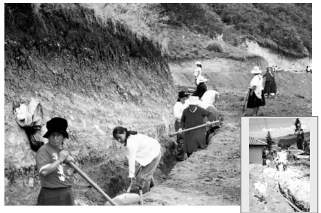
SIGSIG PILOT PROJECT Construction of the Irrigation channel by Minga activity.
