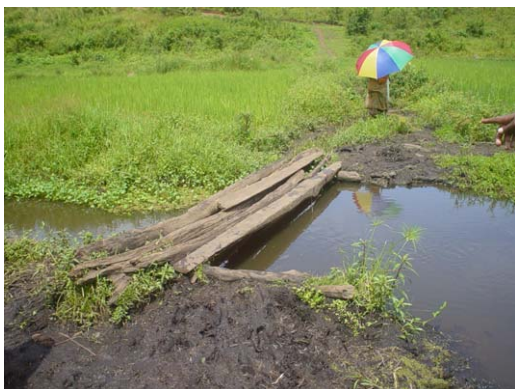
Existing bridge at main channel
