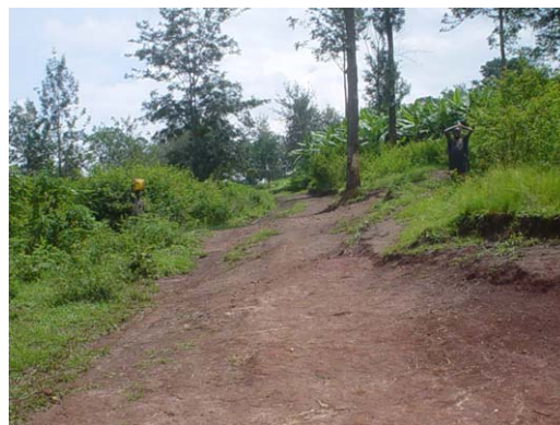
Existing earth road with inclined
