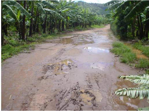
Top soil flow into the farm land
