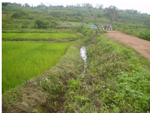
Existing irrigation channel
