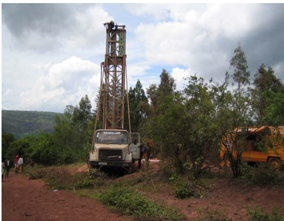
Test drilling, Cyarubare District
