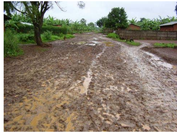
Bad condition of a rural road
