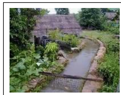
Stone Masonry Canal with Screen
