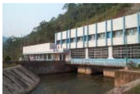
Powerhouse and Tailrace of Nam Dong Hydropower Station
