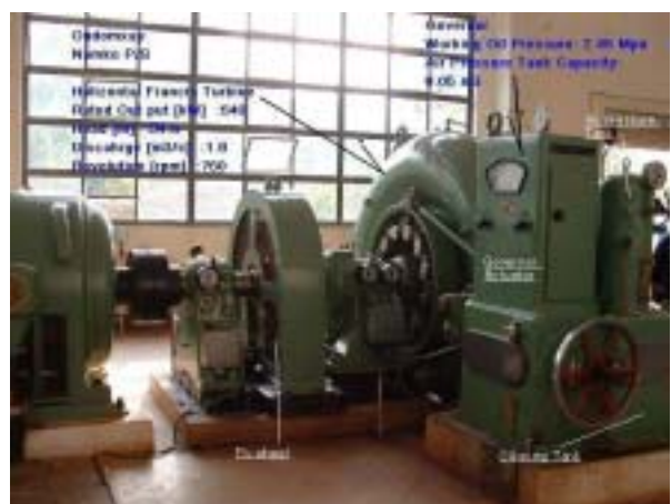
Francis (H) Turbine (500 kW x 3) at Nam Ko HPP in Laos
