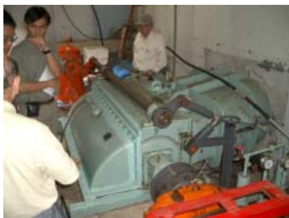
Cross Flow Turbine at Hoshino-Onsen SHP (left: No.1, 50 kW / right: No.3, 50 kW)
