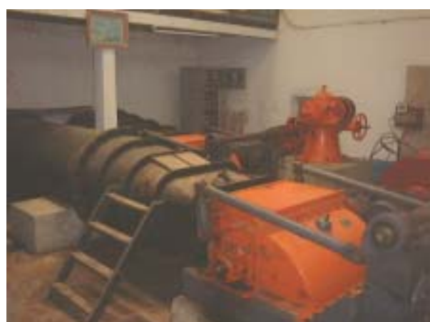
Cross Flow Turbine (90 kW x 2) at Nam Ham Project
