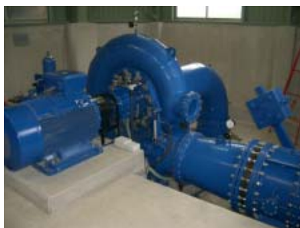
Francis (H) Turbine (132 kW) at Yamaichi SHP in Japan
