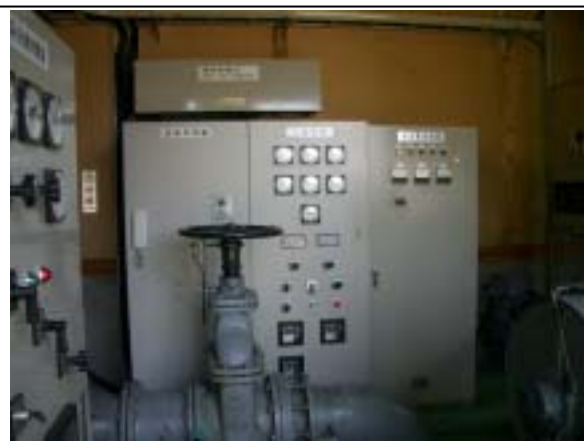
Sluice Valve (left: Trongsa SHP in Bhutan, right: Maguse-Onsen SHP)
