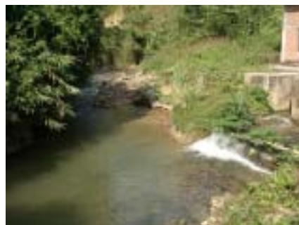
Tailrace of Houay Kaseng Hydropower Station
