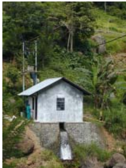
Powerhouse and Tailrace
