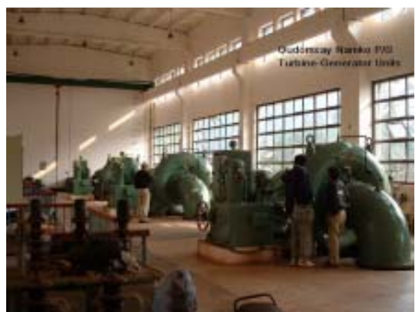
Francis (H) Turbine (500 kW x 3) at Nam Ko HPP in Laos
