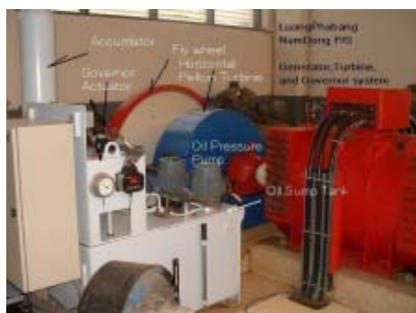
Pelton (H) Turbine (336 kW x 3) at Nam Dong HEPP in Laos
