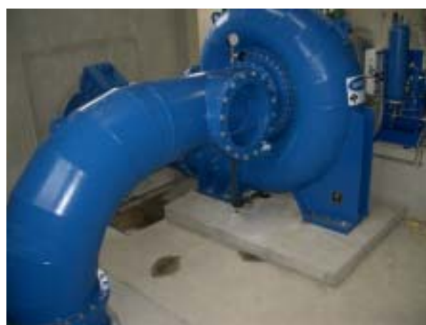
Francis (H) Turbine (132 kW) at Yamaichi SHP in Japan
