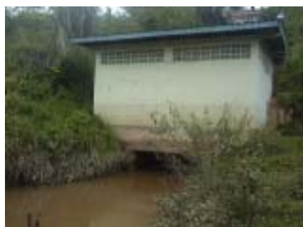
Powerhouse of Nam Ham Hydropower Station
