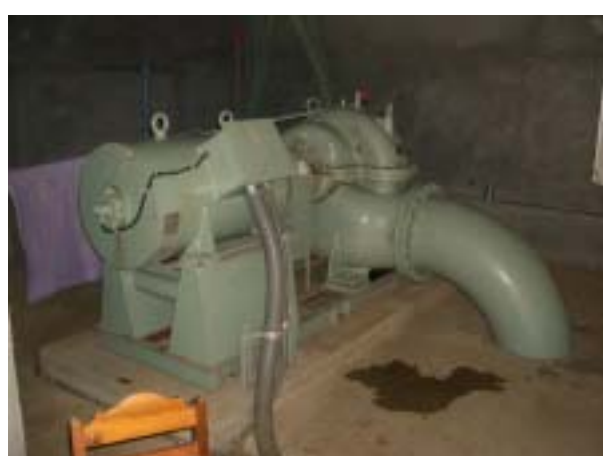
Reversible Pump Turbine (70 kW) at Nam Mong SHP in Laos
