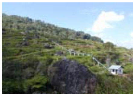
Open Type Penstock
