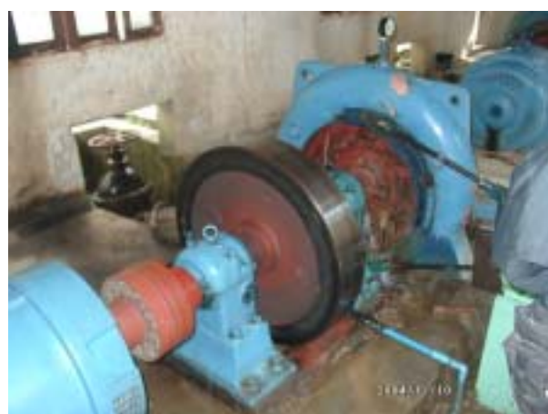
Francis (H) Turbine (155 kW) at Houay Kaseng HPP in Laos
