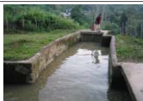
Intake Gate into Penstock of Houay Nung Hydropower Station
