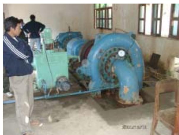
Francis (H) Turbine (155 kW) at Houay Kaseng HPP in Laos
