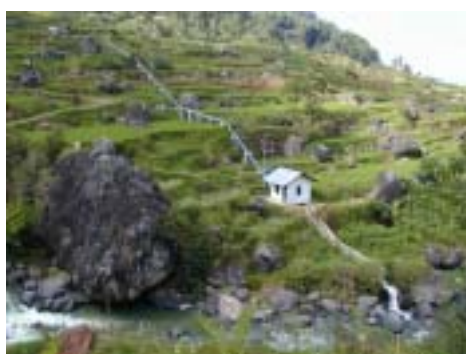
Powerhouse and Tailrace
