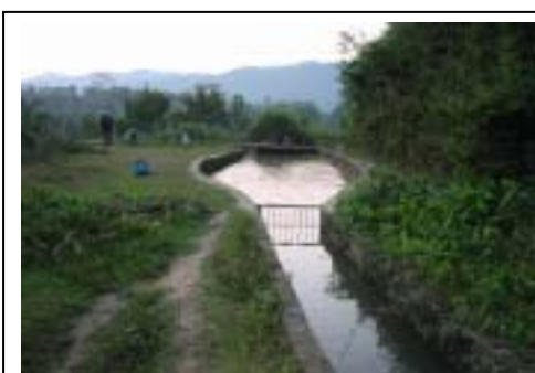
Head Tank of Houay Nung Hydropower Station, Nale, Loungnamtha
