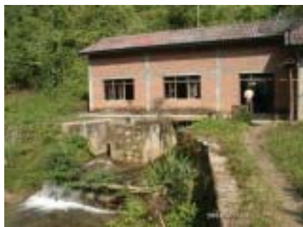
Powerhouse of Houay Kaseng Hydropower Station
