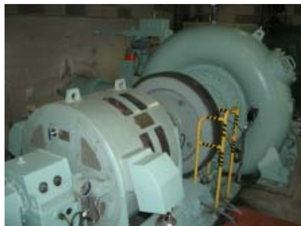
Francis (H) Turbine (150 kW) at Hoshino-Onsen No.2 SHP in Japan
