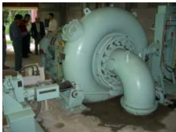
Francis (H) Turbine (150 kW) at Hoshino-Onsen No.2 SHP in Japan
