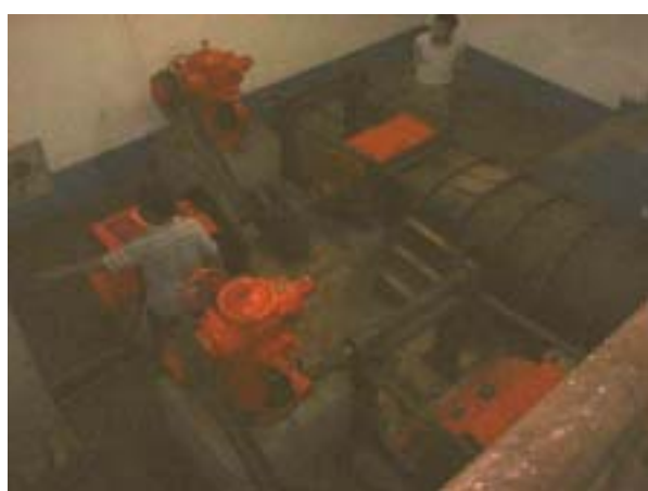
Cross Flow Turbine (90 kW x 2) at Nam Ham Project
