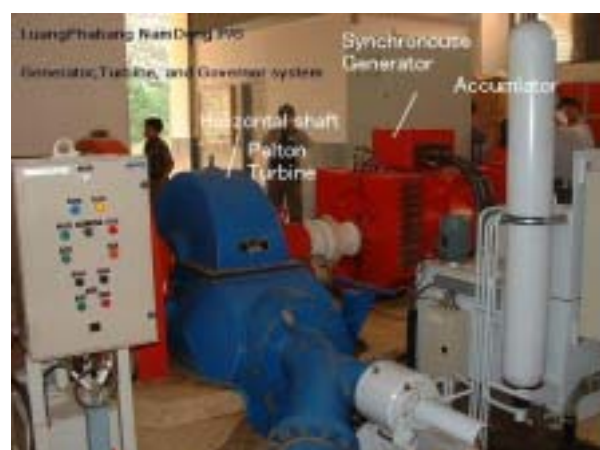
Pelton (H) Turbine (336 kW x 3) at Nam Dong HEPP in Laos
