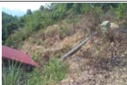
Penstock of Open Type
