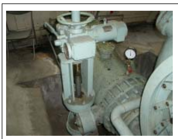
Butterfly Valve in Yukawa No.2 SHP in Japan
