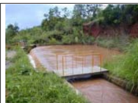
Head Tank with Spillway
