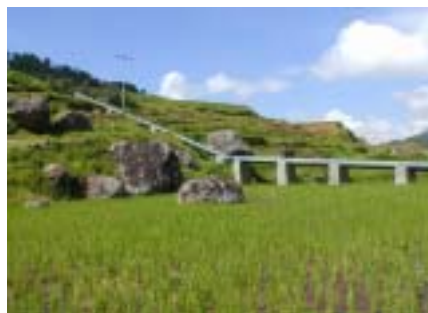
Penstock of Open Type
