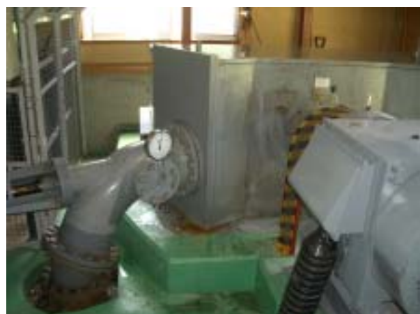
Turgo Impulse Turbine in Maguse-Onsen SHP (95 kW)
