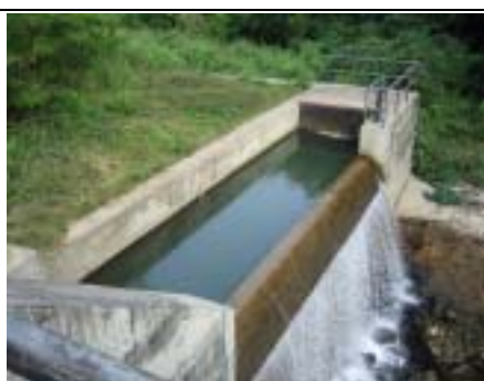
De-silting Basin with Side Spillway (Nam Mong Hydropower Station)
