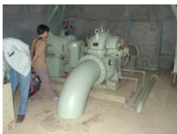
Reversible Pump Turbine (70 kW) at Nam Mong SHP in Laos
