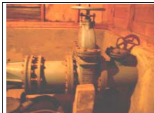
Sluice Valve (left: Trongsa SHP in Bhutan, right: Maguse-Onsen SHP)
