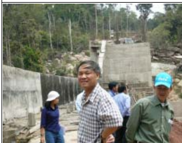
Photo-11 (March 05, 2004) Nam Mang 3 Hydropower Construction Site Visit
