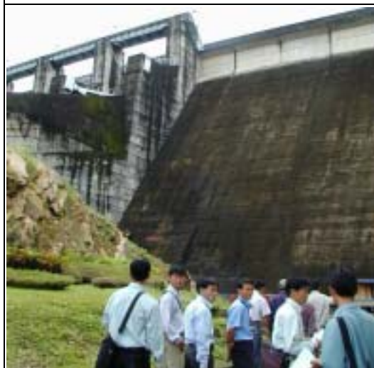
Photo-11 (July 21, 2004) Visit the dam site of Nam Ngum Power Station
