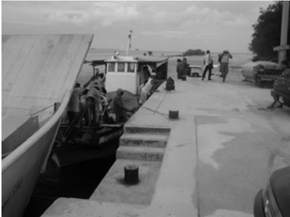
Corrosion of metal portion of Bitts
