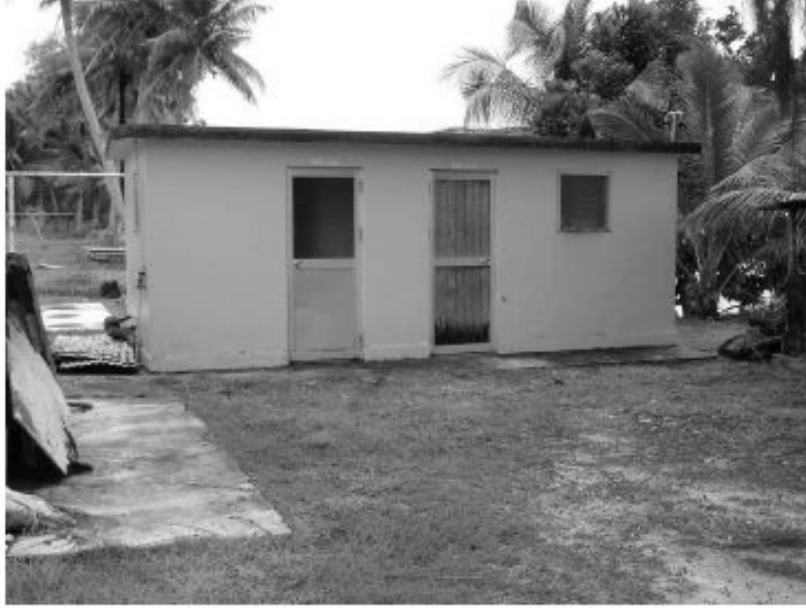
Shed in Land Survey Site 2
