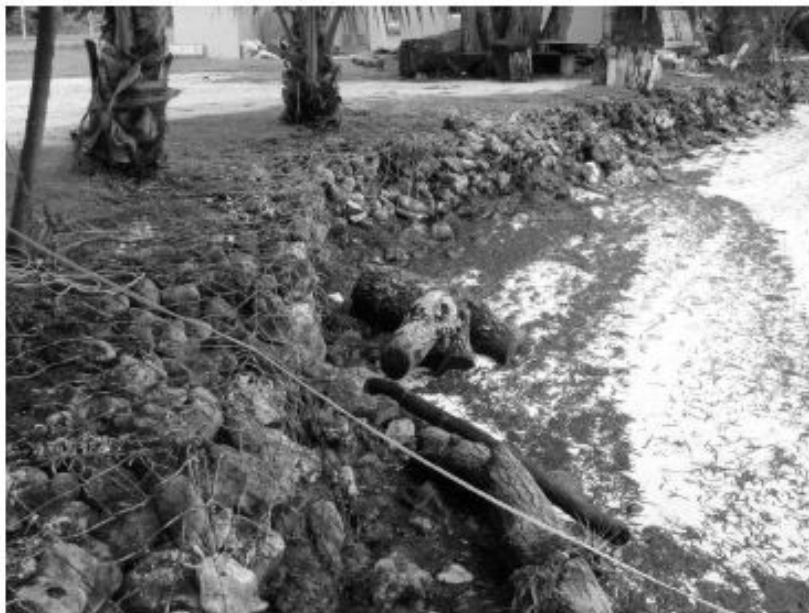
Gabion Sea wall in Land Survey Site 2
