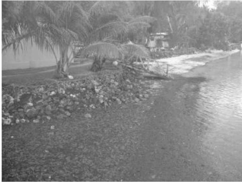
Gabion Sea wall in Land Survey Site 2
