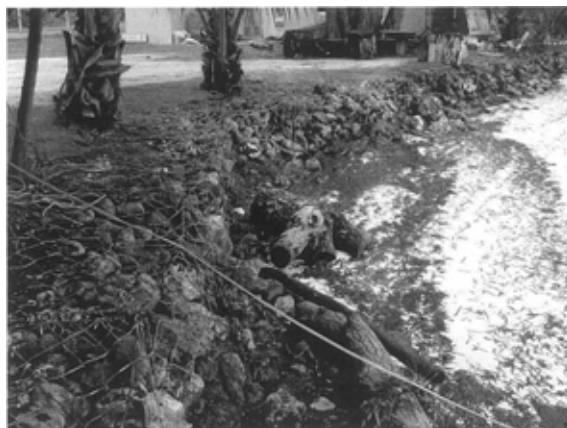
Photo 2.1.3(2)-7 Gabions in West Coast of North Dock
