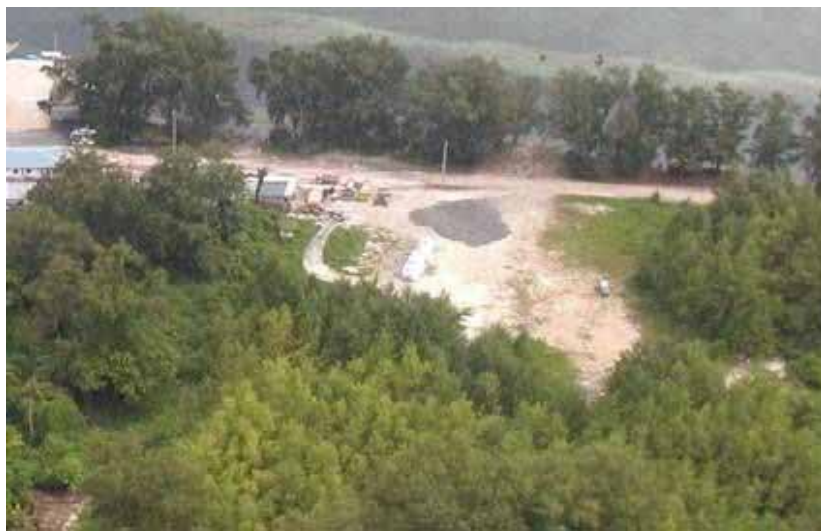
Prospective Site for Temporary Construction Yard
