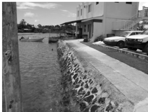
Photo 2.1.3(2)-23 Example of Sloping Revetment with Concrete Masonry
