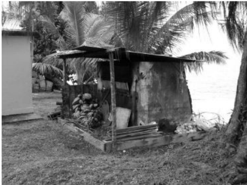
Furnace in Land Survey area Site 2
