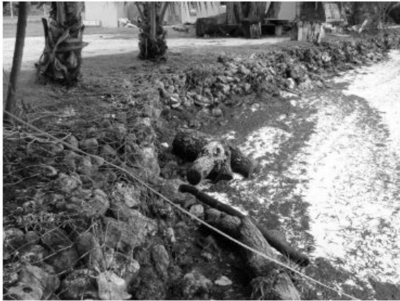
Gabion Sea wall in Land Survey Site 2
