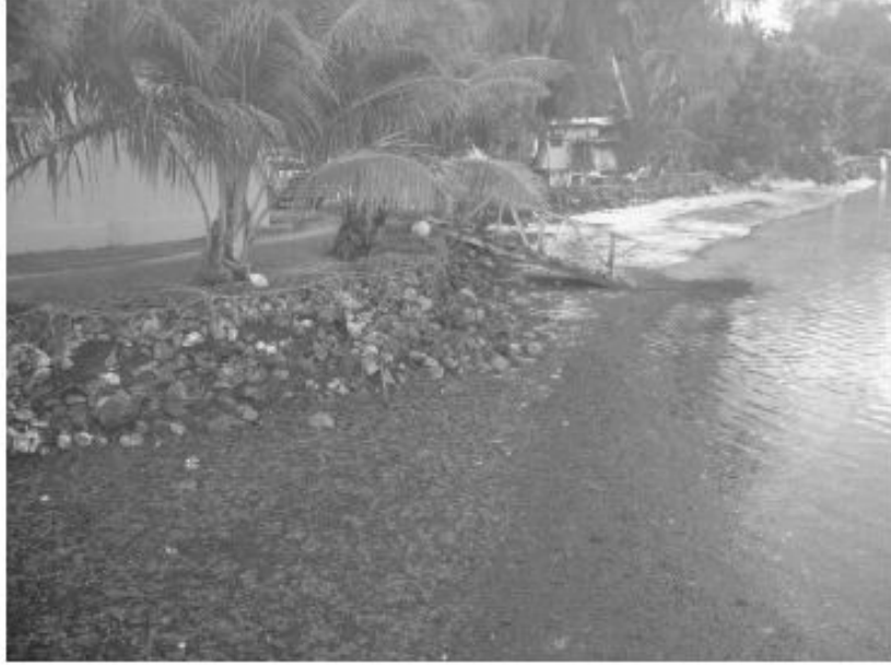
Gabion Sea wall in Land Survey Site 2
