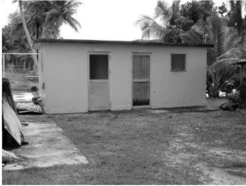
Shed in Land Survey Site 2
