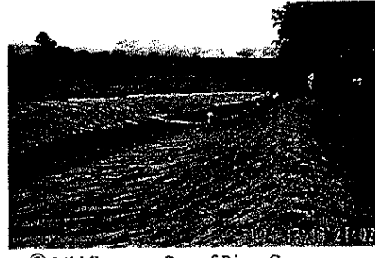
③ Middlestream Part of River Course Changing Works (2004.12)
