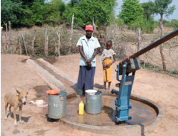
A borehole water supply system using a hand pump, which was constructed under the project (Project for Rural Water Supply in Binga District in Zimbabwe)
