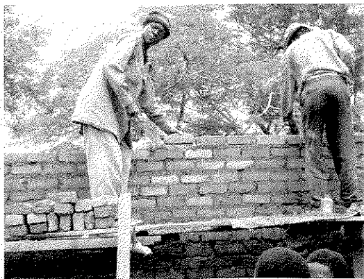
Community people helped school for construction in Nkhata Bay
