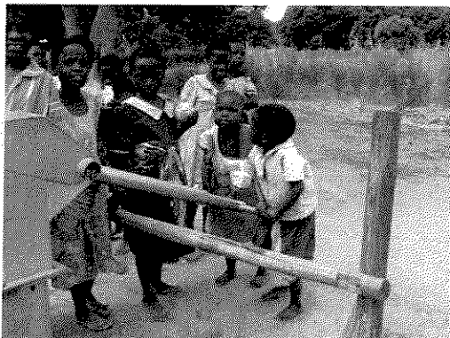
Photo-23: Borehole Construction (Machinga)
