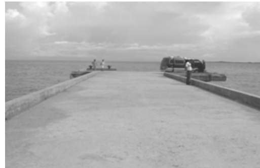
50 m Open Pier
