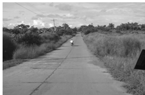
Paved Portion of Access Road
