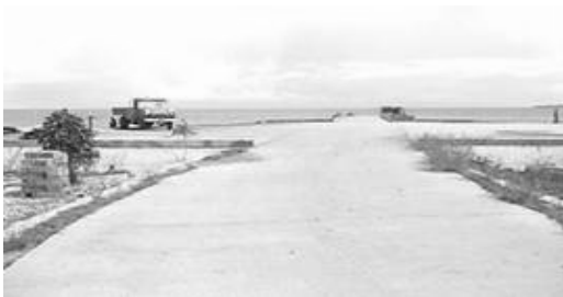
Paved 50 lin.m. access road from the highway to the Port
