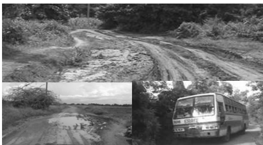
Unpaved portion of access road to Balud Port
