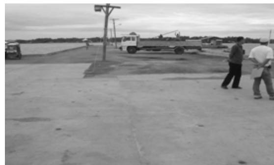
Existing reclamation area (80mx40m). Additional back-up area needed to separate operation area for banca vessels.
