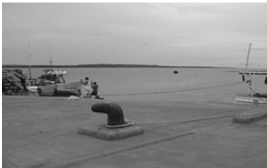
Existing RoRo Ramp. Dredging not needed at RoRo and Pier Berthing Areas. Existing depth of said areas ranges from (-) 5.0m to (-) 8.0m.
