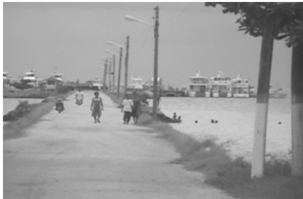
Short macadam road access road, needs concreting (<1km)
