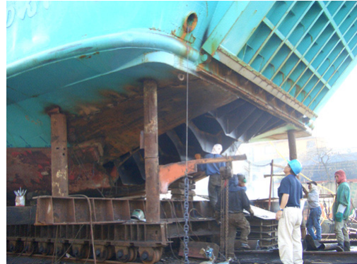
Painting Works at Elfa Shipyard
