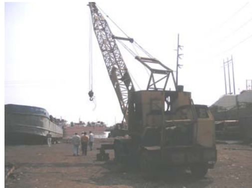
Mobile Crane at Dansyco Shipyard
