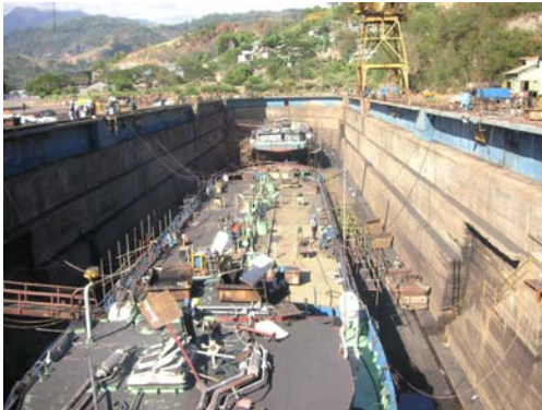
Herma Shipyard's Graving Dock
