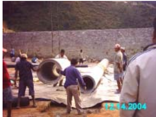
C-2: Leachate Collection Pipes Installation at Sisdol Landfill (December, 2004)
