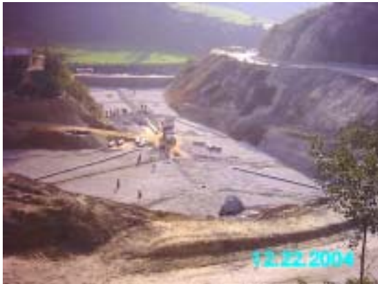
C-2: Drainage Carpet Work at Sisdol Landfill (December, 2004)
