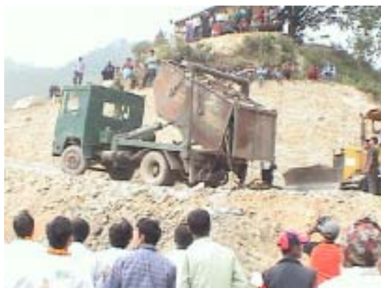
C-2: Commencement of Waste Disposal at Sisdol Landfill (June, 2005)
