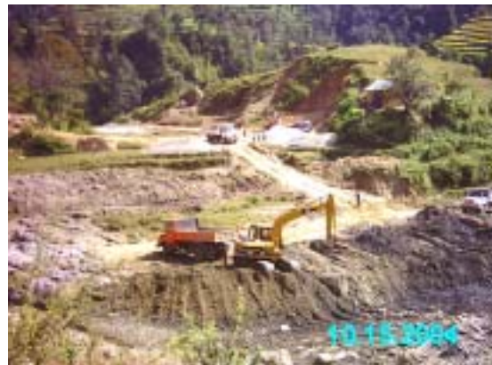
C-2: Excavation Work at Sisdol Landfill (October, 2004)
