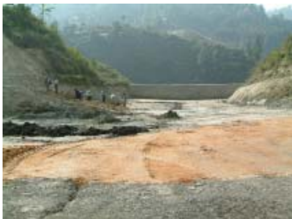
C-2: Clay Liner Work at Sisdol Landfill (November, 2004)
