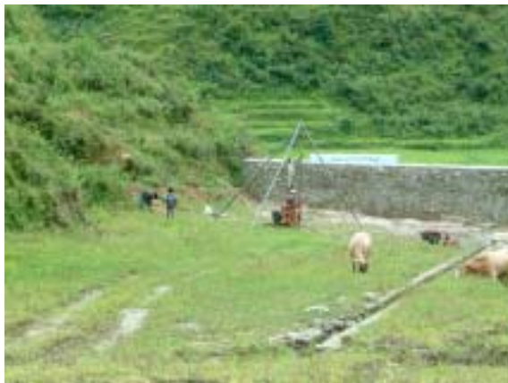
C-2: Soil Investigation in Sisdol (July, 2004)
