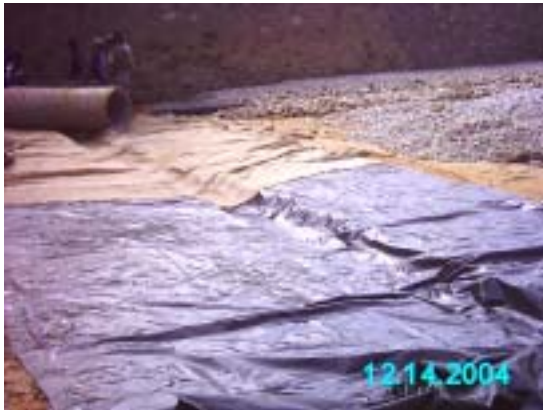
C-2: HDPE Under Main Pipes at Sisdol Landfill (December, 2004)
