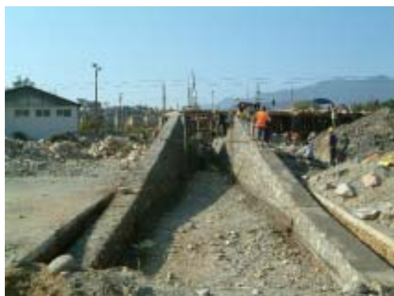
A-3: Construction for Improvement of Teku T/S (November, 2004)
