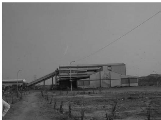
Excel's Composting Facility in Ahmedabad.
