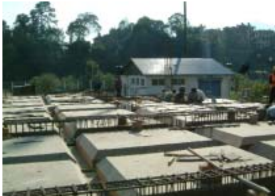
A-3: Construction for Improvement of Teku T/S (November, 2004)
