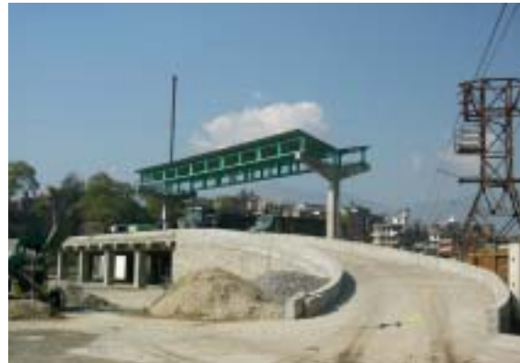
A-3: Completion of Improvement of Teku T/S (March, 2005)
