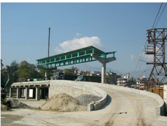
A-3: Completion of Improvement of Teku T/S (March, 2005)
