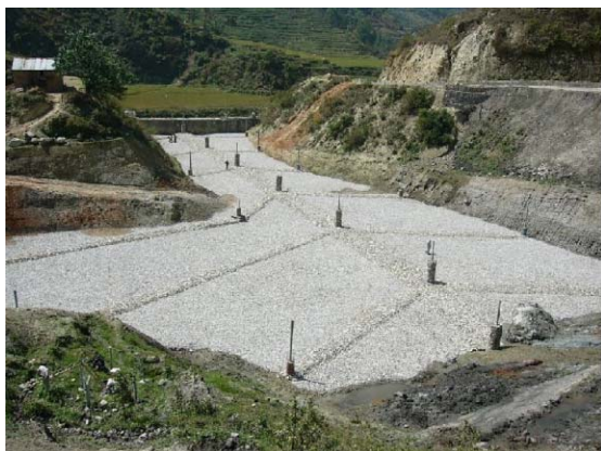
C-2: Completion of Improvement of Sisdol Landfill (December, 2004)
