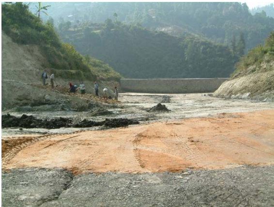
C-2: Improvement of Sisdol Landfill -Clay Liner Work- (November, 2004)
