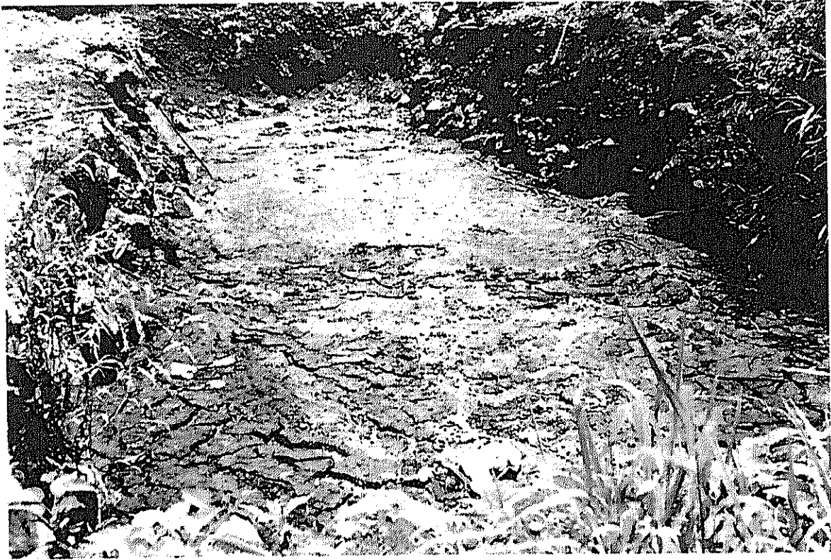
SEPTAGE DISPOSAL PITS
