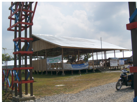
Photo 5. A temporary school in IDPC located at inland area
