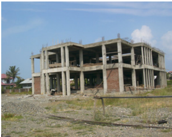
Still under construction since 2002
