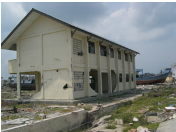
The ruin of Classroom building of SMK4
