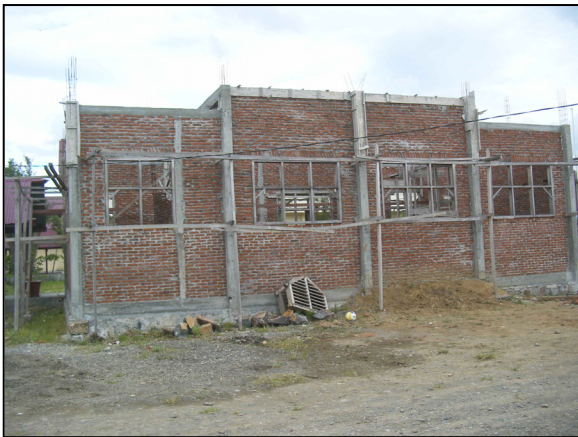
Suspended construction of science laboratory of SMP Percontohan
