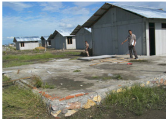
Temporary houses are under construction beside the TK Negeri
