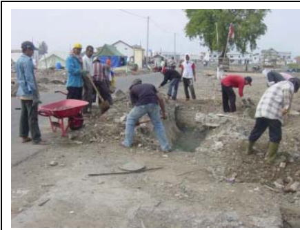
Recovery Work for Digging Channels, Kuta Raja Region
