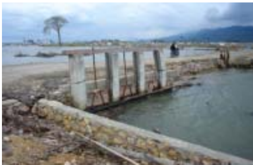
Drainage channel at Iskandal Mudah
