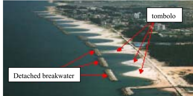
Figure 4.9.6 A series of Detached Breakwater
