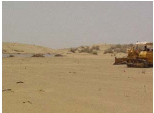
Bulldozer under the jurisdiction of the Sukkur Subdivision office, plowing the desert
