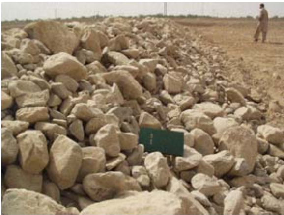
Embankment made from stones collected during the reclaiming process above; retains rainwater and protects against soil erosion
