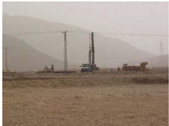
Groundwater drilling (performed by the Power and Irrigation Department)
