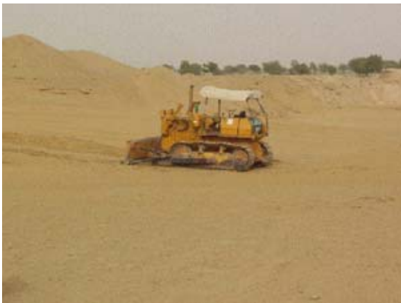
Bulldozer under the jurisdiction of the Bahawalpur District office, developing farmland at an altitude of about 3 meters for water retention
