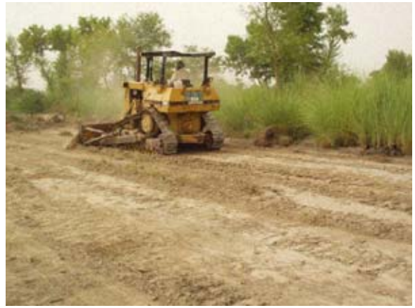
Bulldozer preparing for a fishpond (under the jurisdiction of the Faisalabad District office)
