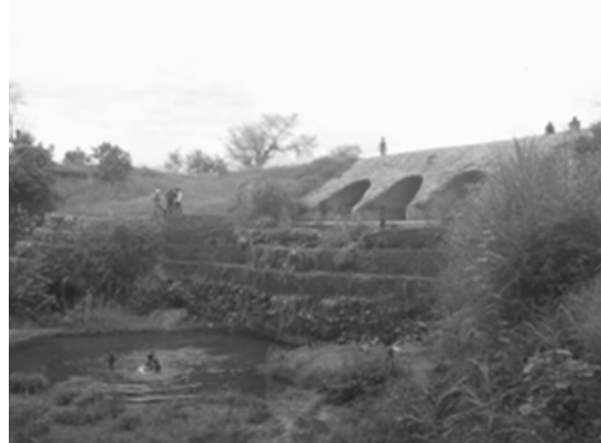
Picture 2-1 : Angoni Culvert
