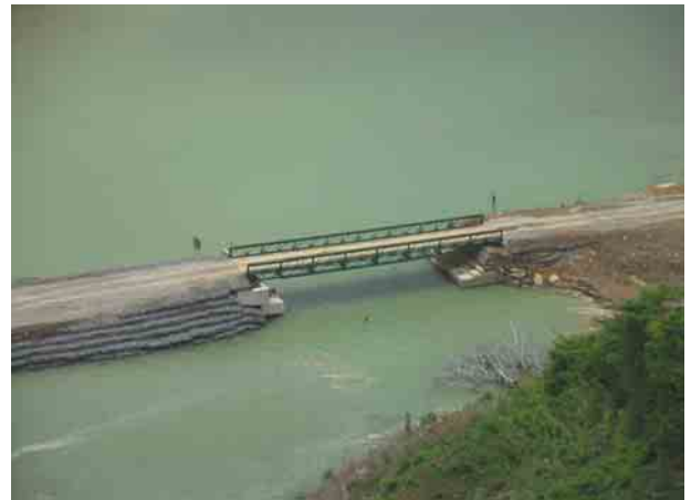
KM 27+840 Peulot Bridge (bailey+gabion protection)
