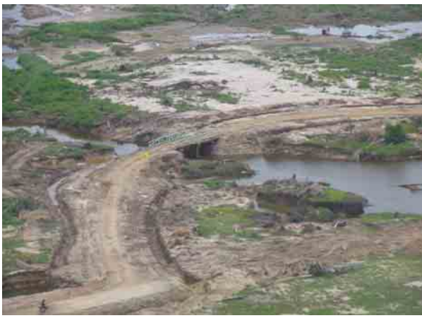
KM 164+540 Bakong 1 Bridge (west coast road) (Reconstruct with concrete bridge along straight alignment)
