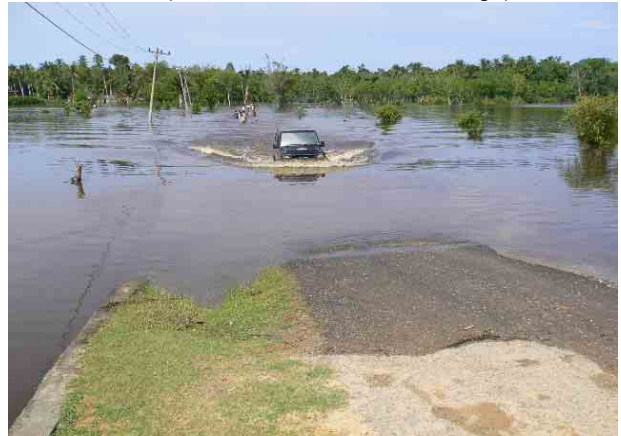
KM 251+000 (original village road, flood section) (Raise road by embankment and AC pavement)
