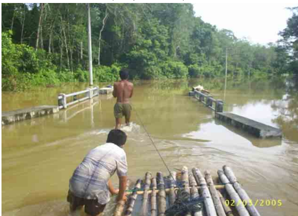
KM 246+800 (original village road, flood section) (Raise road by embankment and AC pavement)
