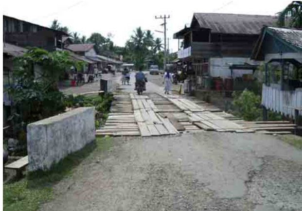
KM 236+183 Kureung Wayla Bridge (original village road) (Reconstruct with concrete bridge)
