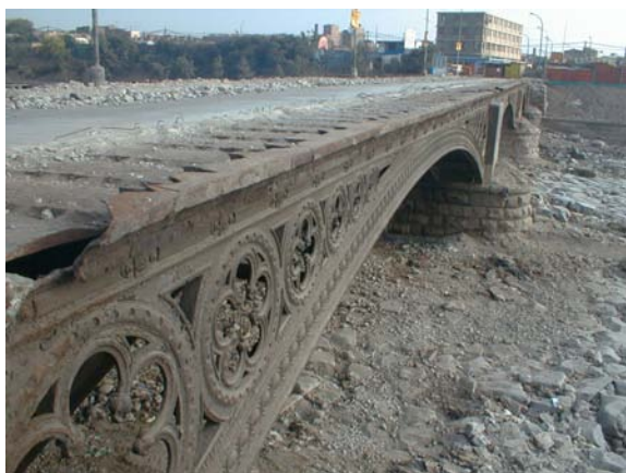
Balta Bridge at Rimac River (Lima District)
