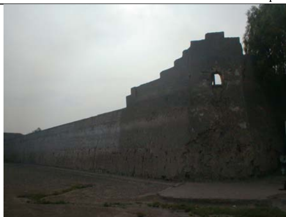
City Wall Watch Tower (El Agustino District.)
