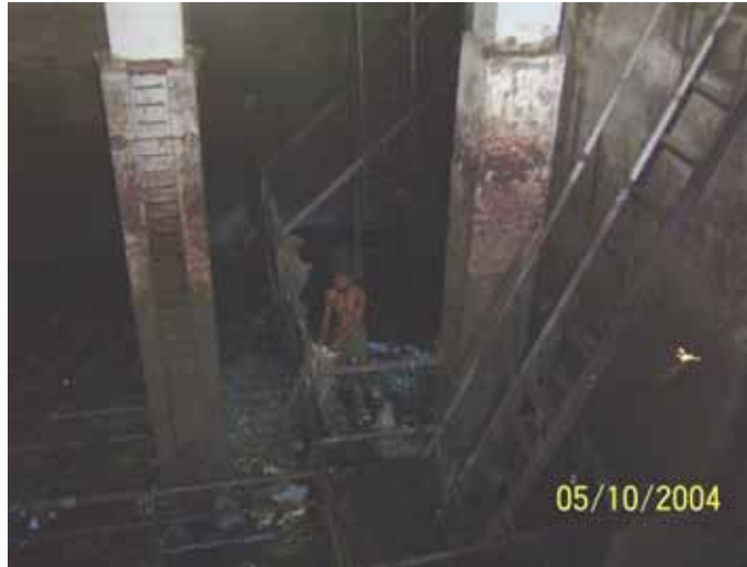
Wet Sump at Alopibagh SPS (Manual Collection of Screenings)
