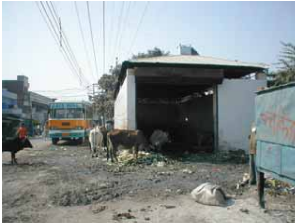
Photo 2.6 Roofed-Type Secondary Collection Depot along GT Road
