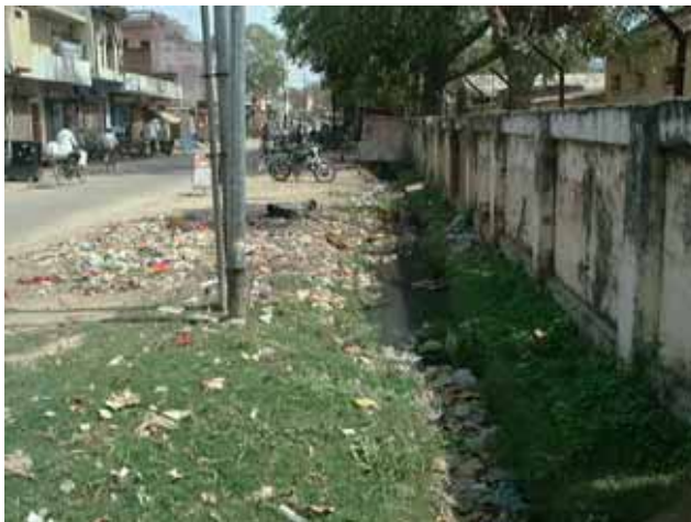
Photo 4.2 Condition of Small Street Gutter
