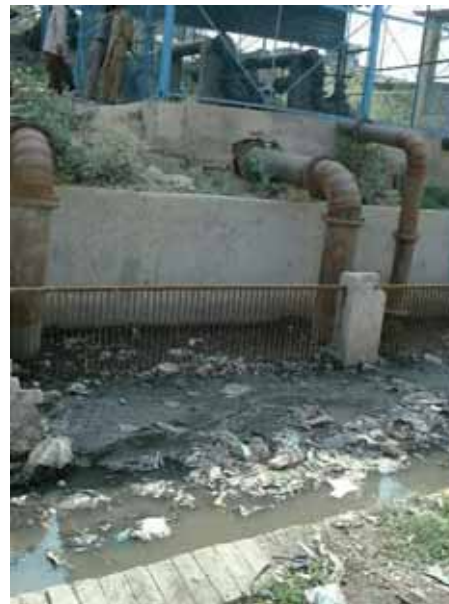
Photo 4.3 Drainage Pump Station
