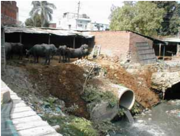
Photo 6.6 Excrements Flowing into Nala from a Cattle House (Wazirganj Nala, Lucknow)
