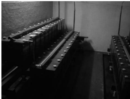
Battery of Control and Communication Equipment
