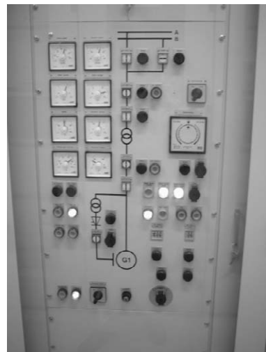
Control Board of Gen & Tr.
