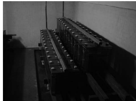
Battery of Control and Communication Equipment
