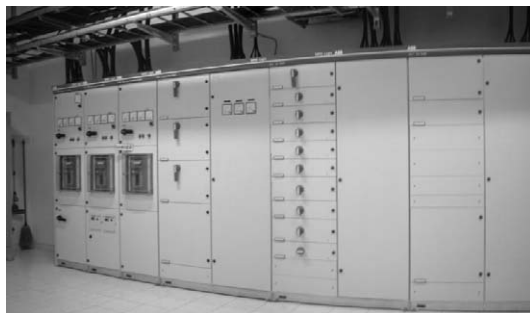
Station Service Cub. & Unit 1 & 2 Motor Control Center (MCC)
