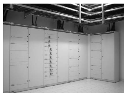
Station Service Cub. & Unit 1 & 2 Motor Control Center (MCC)
