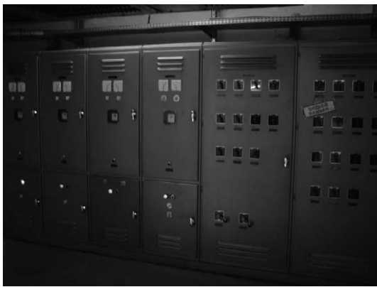
Auxiliary control board (NFB and ACB)
