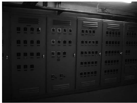
Auxiliary control board (NFB and ACB)
