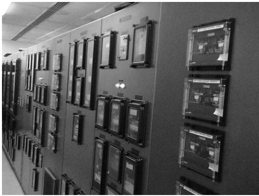
Protection relay boards and renewed lockout relay # 86
