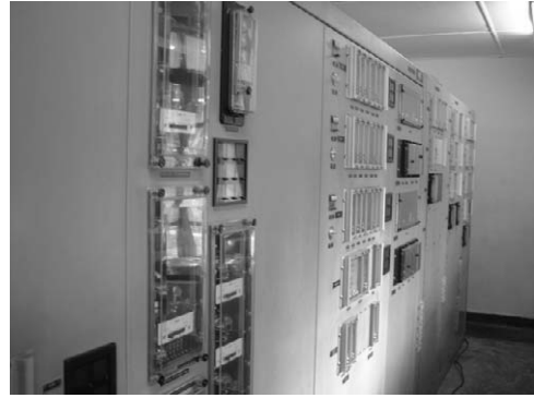
3.3 kV Switchgear & Distribution Line Control and Protection Relay Boards
