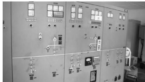
3.3 kV Switchgear & Distribution Line Control Boards
