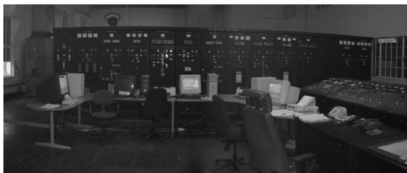
Computer control with CRT (Old boards <black color>)
