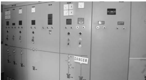
3.3 kV Switchgear & Distribution Line Control Boards
