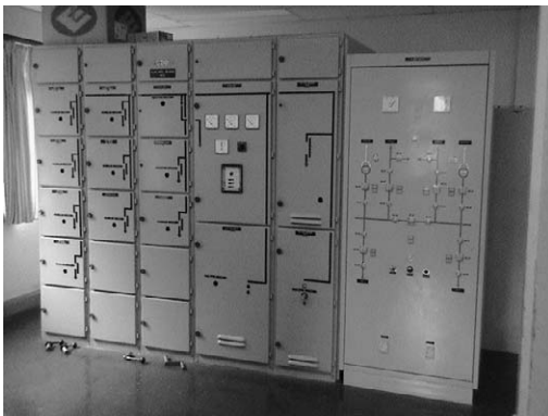
Motor Control Centers for Unit 1 & 2
