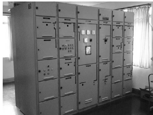
Motor Control Centers for Unit 1 & 2
