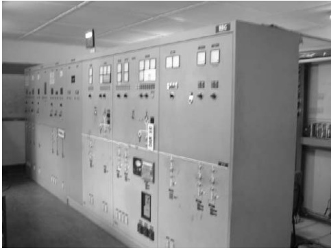
3.3 kV Switchgear & Distribution Line Control and Protection Relay Boards
