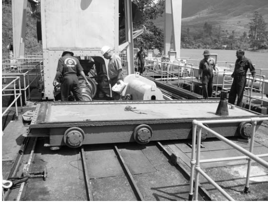
Picture 6.3 Repairing of Intake Equipment
