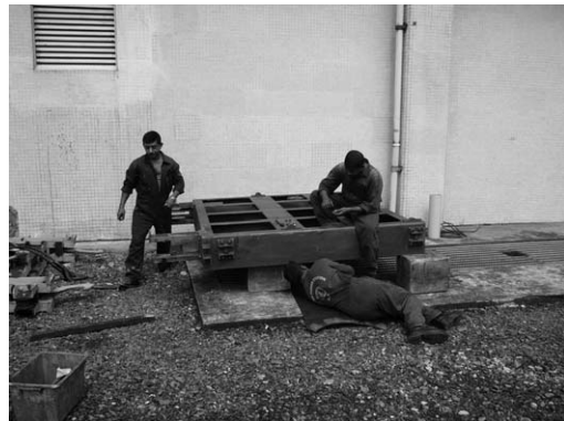
Picture 6.14 Repairing the tailrace gate by CEB
