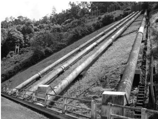
Picture 6.5 Panorama view penstock
