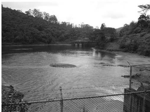
Picture 6.19 Sedimentation of reservoir
