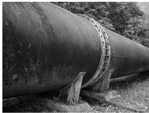
Picture 6.22 Mechanical joint
