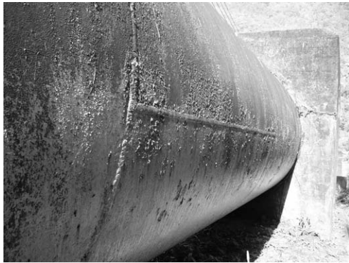
Picture 6.23 Outside surface of welded joint
