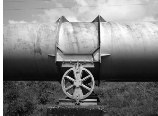
Picture 6.2 Ring girder support with wheels
