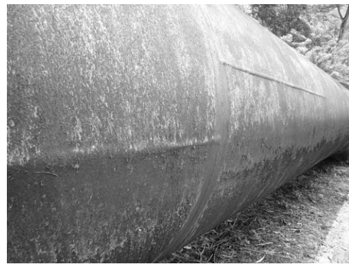
Picture 6.16 Touch up paint for welding joint by CEB
