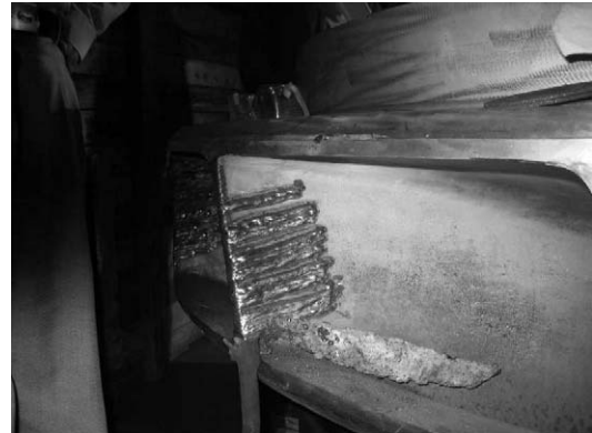
Picture 7.9 Repair Welding of Polpitiya Runner
