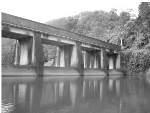
Picture 6.9 Spillway of Norton Dam
