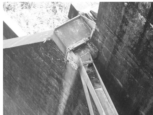
Picture 6.26 Arm requires drain holes
