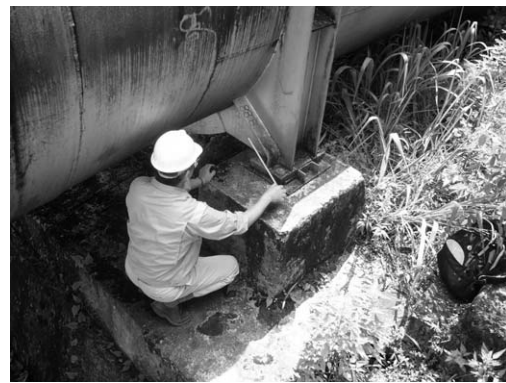
Picture 6.11 Check of slide shoe
