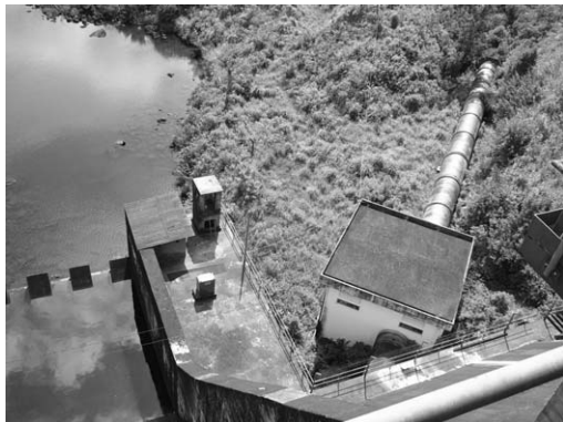
Picture 6.13 Intake guard valve house
