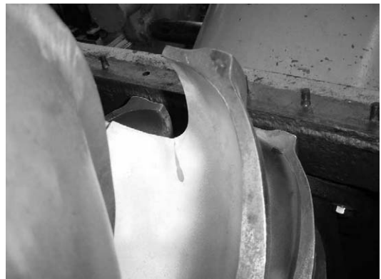
Picture 7.6 Indication of Runner Crack at Old Laxapana Stage I
