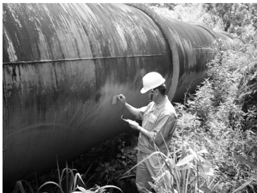
Picture 6.10 Measuring for plate thickness
