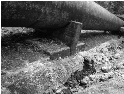
Picture 6.17 Repair work of drain
