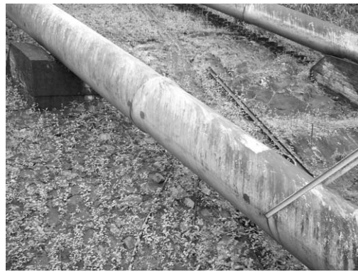
Picture 6.6 Spigot & socket (1 st stage)
