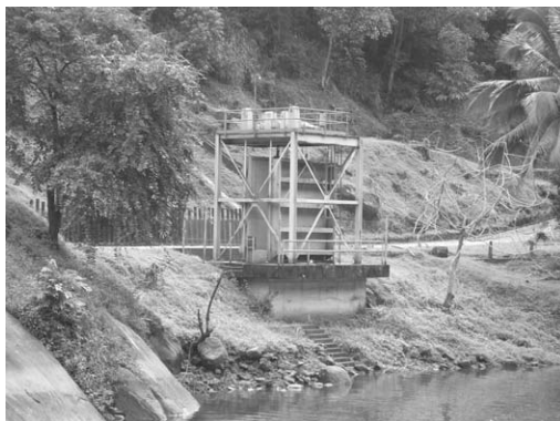
Picture 6.29 Intake equipment
