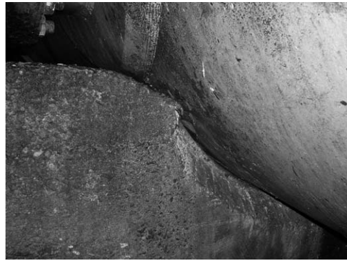
Picture 6.18 Filler material of concrete saddle
