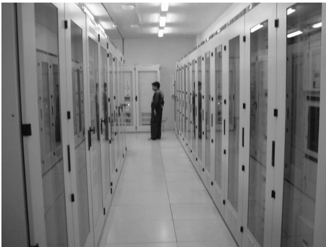
Control Boards of Generator / Transformer (left site) and Transmission Line (right side)
