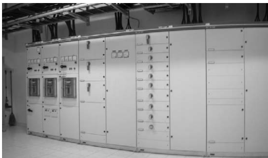
Station Service Cub. & Unit 1 & 2 Motor Control Center (MCC)
