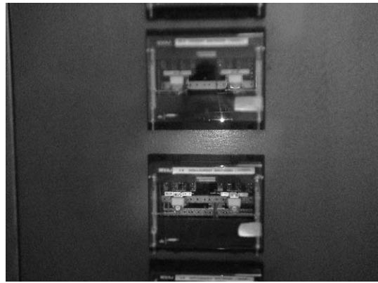
Protection relay boards and renewed lockout relay # 86
