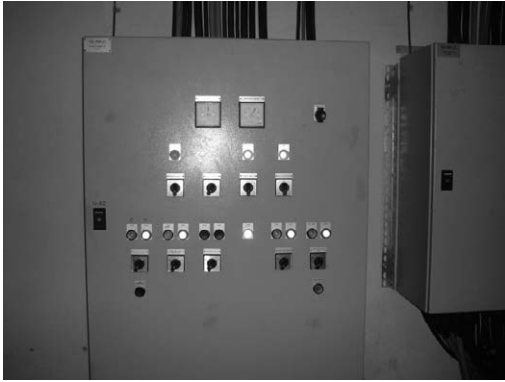
Control Panel of Turbine (left ) and Generator Auxiliary Equipment (right)
