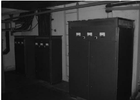
Battery charger of control & communication
