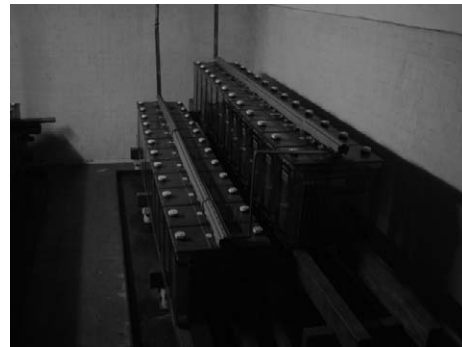
Battery of Control and Communication Equipment
