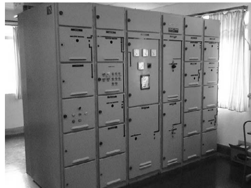
Motor Control Centers for Unit 1 & 2
