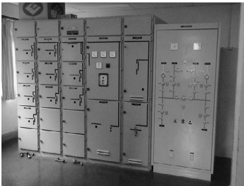
Motor Control Centers for Unit 1 & 2
