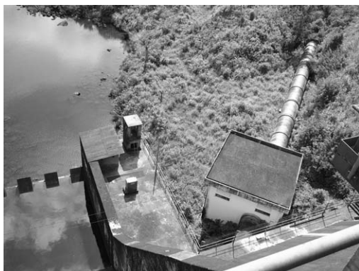
Picture 6.13 Intake guard valve house
