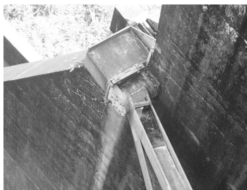
Picture 6.26 Arm requires drain holes
