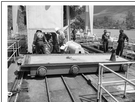
Picture 6.3 Repairing of Intake Equipment
