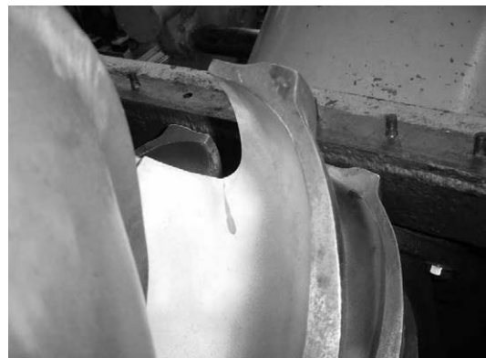
Picture 7.6 Indication of Runner Crack of Old Laxapana Stage I
