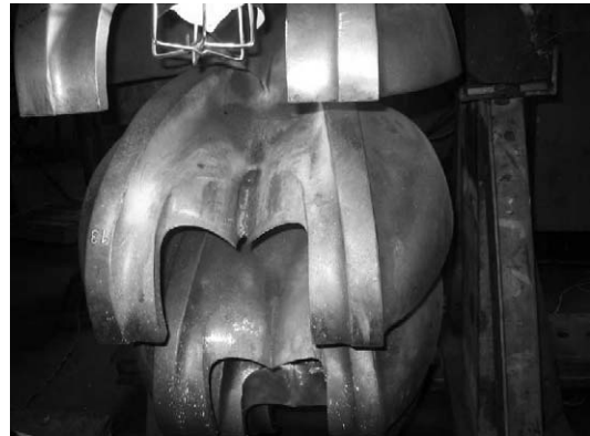
Picture 7.4 Repairing of Runner Crack of Old Laxapana Stage I
