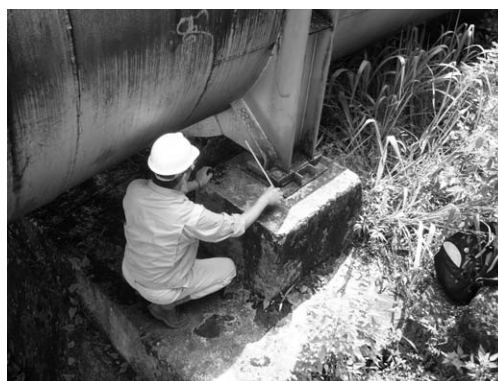
Picture 6.11 Check for slide shoe
