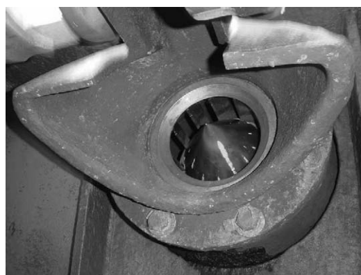
Picture 7.3 Diffuser and Needle of Old Laxapana Stage I
