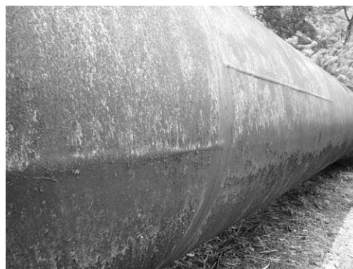
Picture 6.16 Touch up paint for welding joint by CEB
