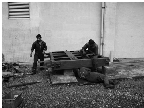
Picture 6.14 Repairing the tailrace gate by CEB
