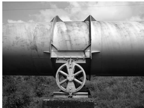
Picture 6.2 Ring girder support with wheels
