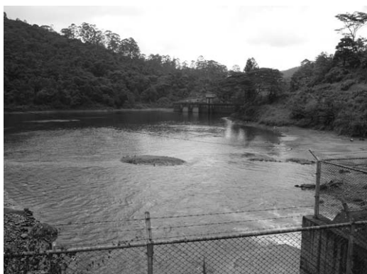
Picture 6.19 Sedimentation of reservoir
