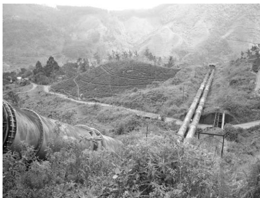
Picture 6.1 Panorama view of penstock
