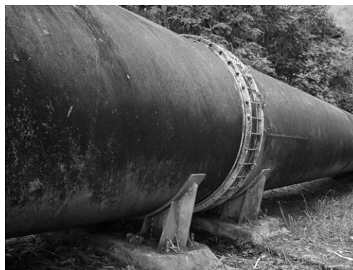
Picture 6.22 Mechanical joint
