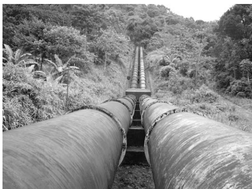
Picture 6.15 Panorama view of penstock
