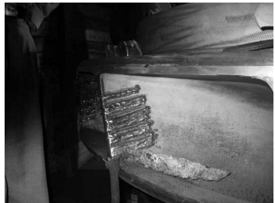
Picture 7.9 Repair Welding of Polpitiya Runner
