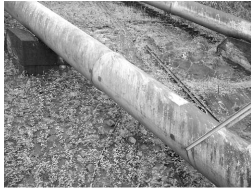
Picture 6.6 Spigot & socket (1 st stage)
