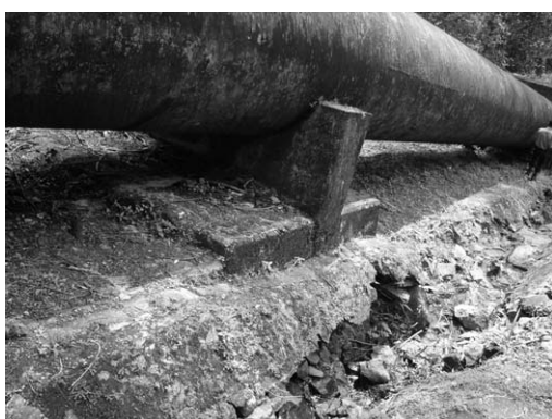
Picture 6.17 Repair work of drain
