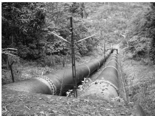
Picture 6.21 Panorama view of penstock
