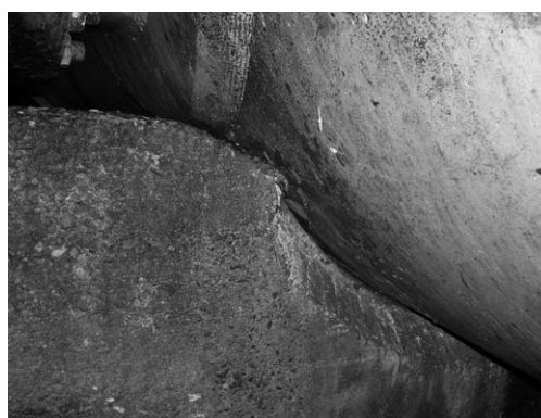
Picture 6.18 Filler material of concrete saddle
