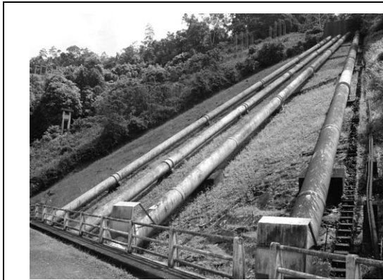
Picture 6.5 Panorama view of penstock
