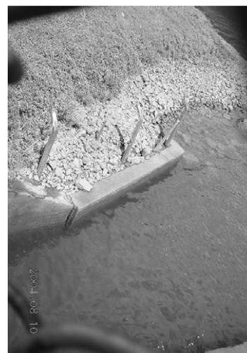
Picture 5.12 Displacement in Retaining Wall at Outlet
