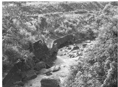
Picture 5.22 Erosion in Concrete Wall
