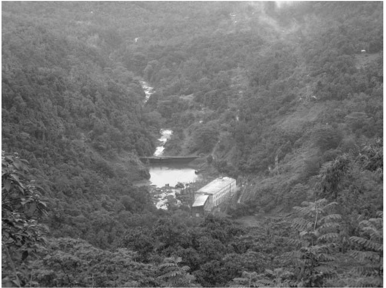
Laxapana Hydropower Station (Old and New Laxapana Hydropower Station)
