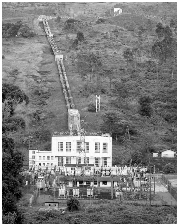
Wimalasurendra Hydropower Station
