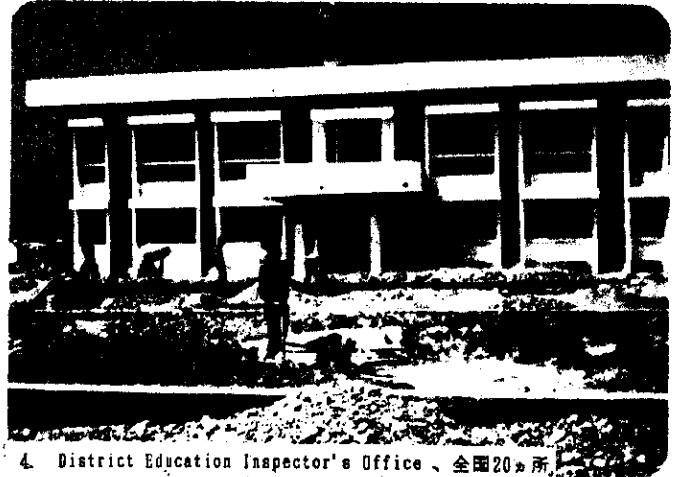
4. District Education Inspector's Office、全国20ヶ所。
