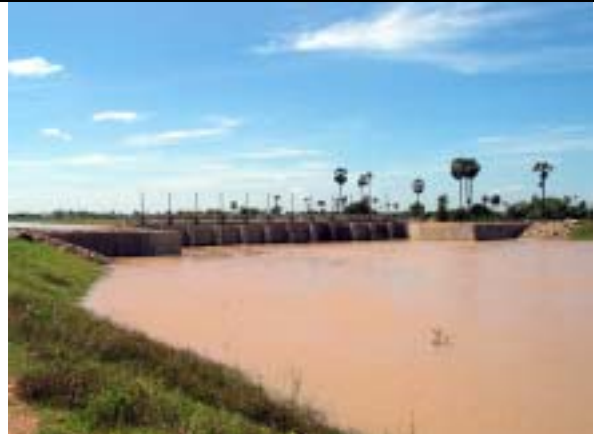
Photo-2: Oct.28, 2003. Flood Relief Channel constructed by ADB emergency flood rehabilitation project in the downstream the Prek Thnot River. The capacity is estimated at 300 m 3 /s.
