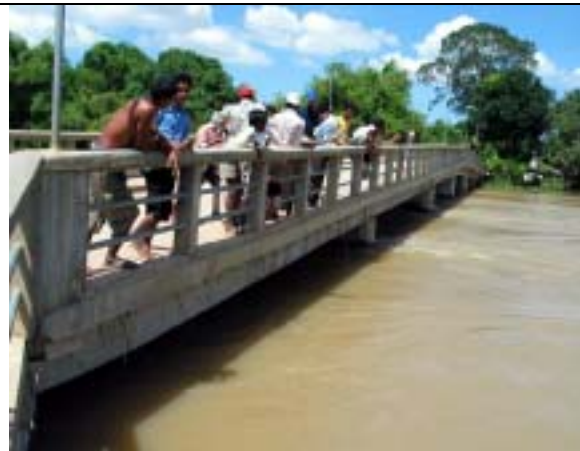
Photo-3: Oct.28, 2003. Prek Thnot River at Kong Noy, Kandal. Measured discharge was 750 m 3 /s. A village on the left bank is inundated. Flood dike on the left bank is located beyond the village.
