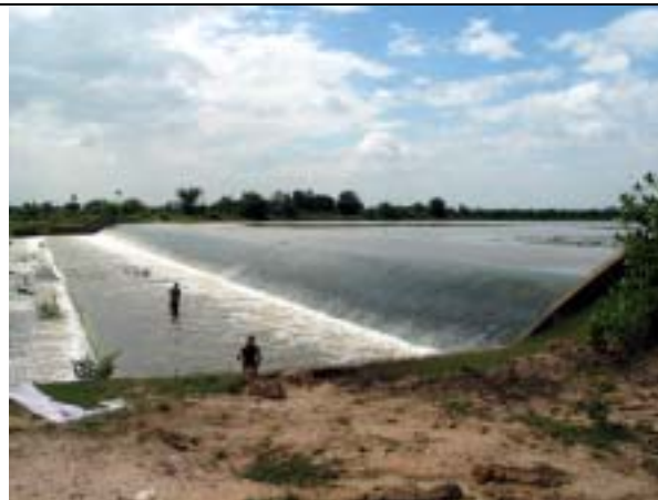
Photo-4: Oct.28, 2003. Spillway of Ou Krang Ambel reservoir on the left bank of the Prek Thnot River. The irrigation system diverts water form a tributary of the Prek Thnot and Roleang Chrey North Main Canal.
