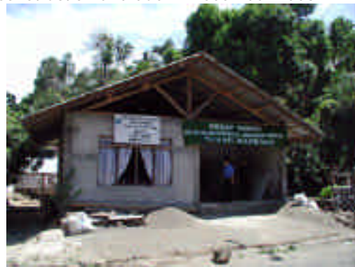
An outside view of the office of village head, which temporarily houses the new school. The white signboard proudly indicates the school's name. The banner on the right, originally made for a REDIP-supported campaign in 2000, is hung here to show the school is affiliated with REDIP2.
