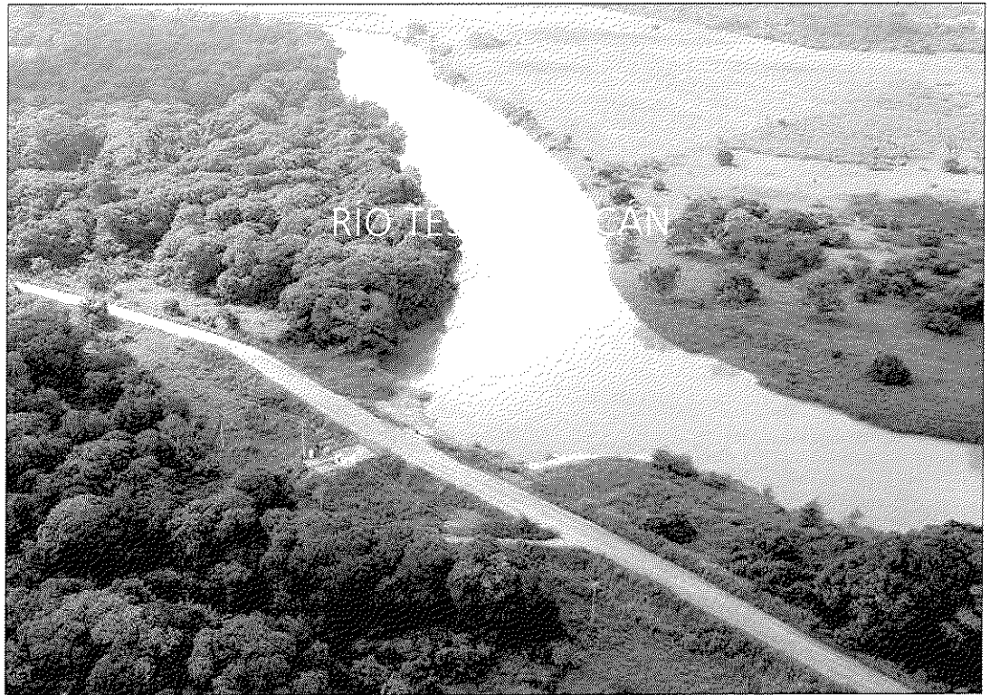
PUMPING STATION IN THE TESECHOACÁN SUBMODULE
