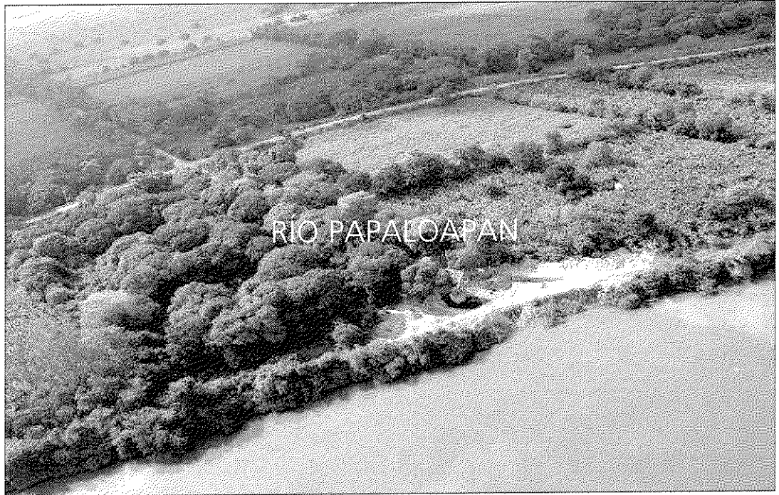
PUMPING STATION IN THE TLACOJALPAN II SUBMODULE
