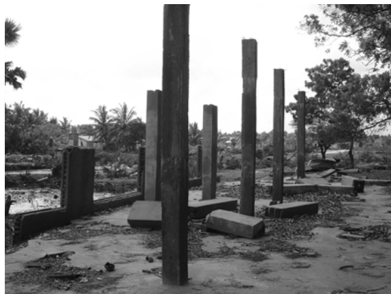
Only some RC columns stood on the ground, Kinniyai (Trincomalee) Tsunami's Force is almost proportional to projective area of column or wall
