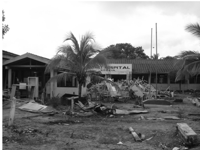
Hospital destroyed, Kinniyai (Trincomalee)
