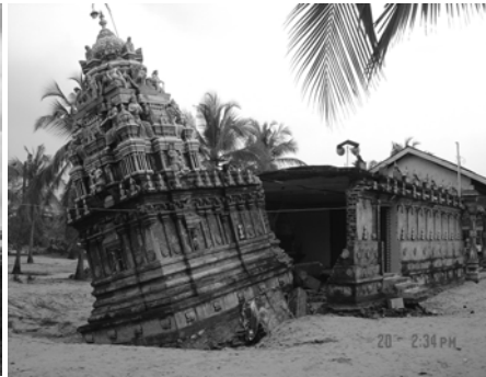
Buddhism temple destroyed, Batticaloa Wall: 3 layer brick: strong Tower: sands around foundation were washed out by Tsunami
