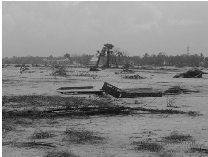
Ground Zero: Tsunami fully washed off everything except a Temple and some trees, Batticaloa
