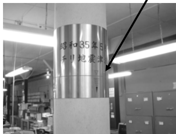
Inundated level by Tsunami is marked on a pillar of the Town Office.
