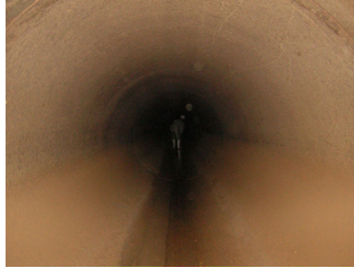
Figure1.19 Inside of Siphon
