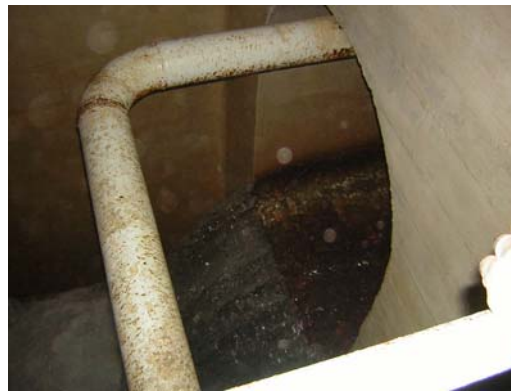
Figure1.10 Condition of the New Reservoir with the Exit of New Tunnel
