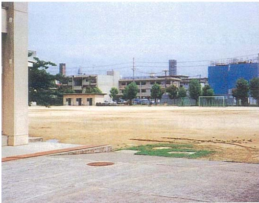
Figure M.2.30 Sample of Stormwater Retention Facility (In School/University Ground)
