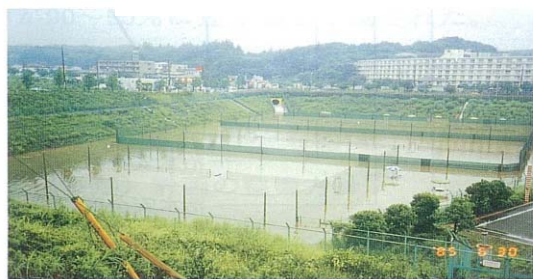
Figure M.2.33 Sample of Stormwater Retention Facility (Tennis Court)
