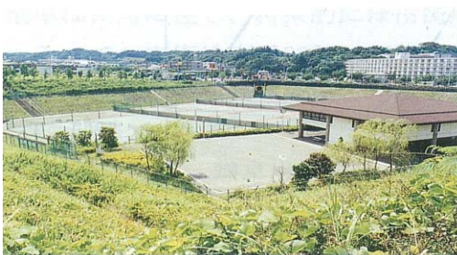
Figure M.2.33 Sample of Stormwater Retention Facility (Tennis Court)
