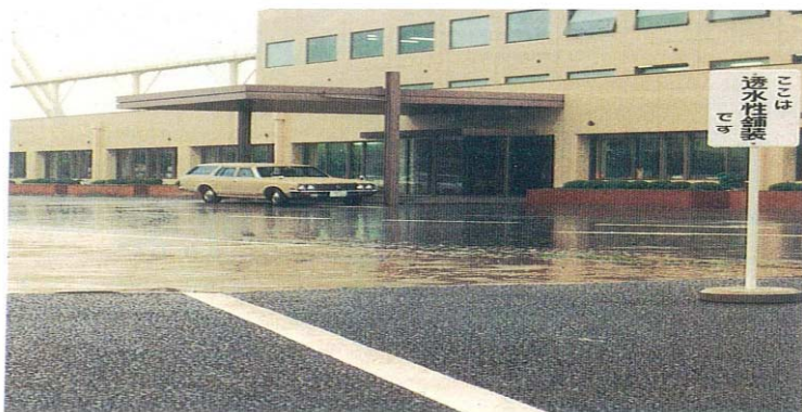
Figure M.2.31 Sample of Stormwater Retention by Permeable Pavement (Parking Area)
