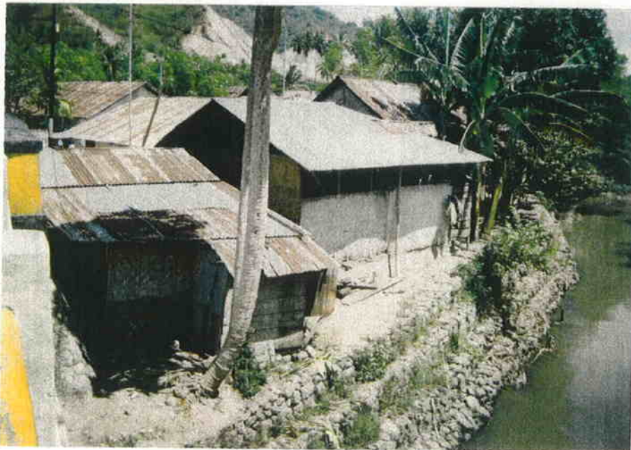
Temporary Structure in House (Stretch II Right, Lower Bolango River Improvement) in Kel. Siendeng (Kotamadya Gorontalo)
