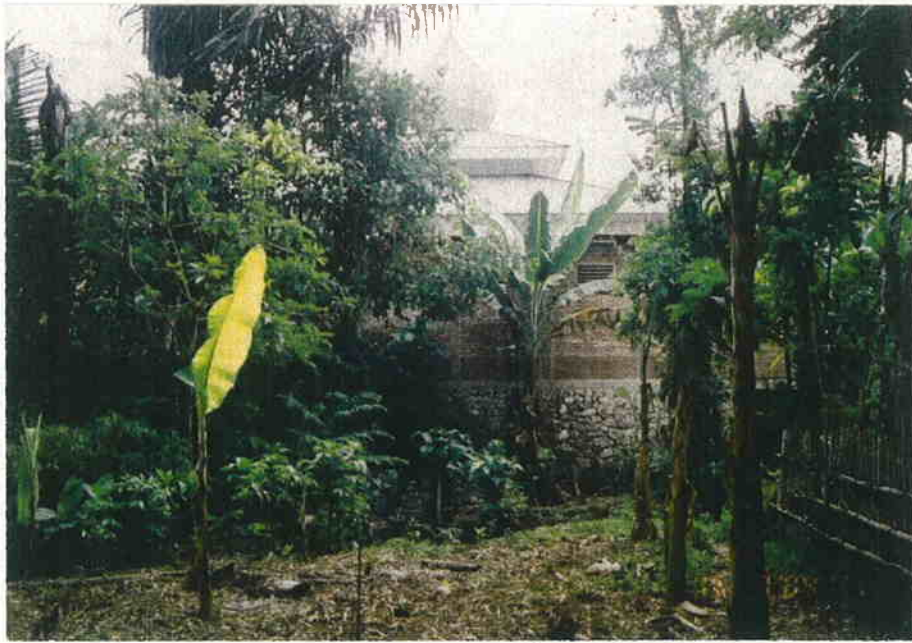
Mosque and Pekarangan around Existing Ditch (Tamalate Floodway) in Kel. Oluhuta (Kab. Bone-Bolango)
