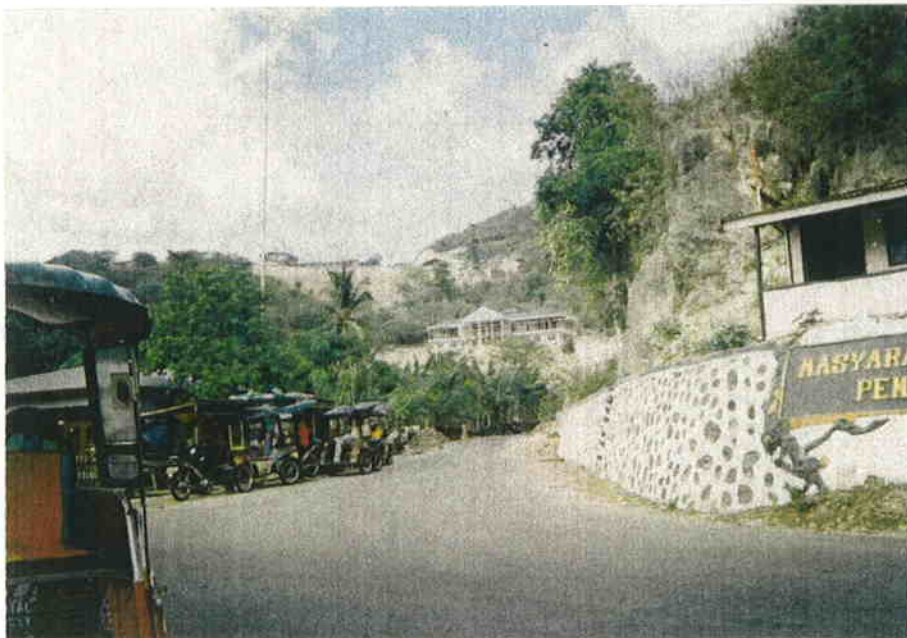
Bentor and the Provincial Authority Buildings under Construction in Kel. Botu (Kotamadya Gorontalo)
