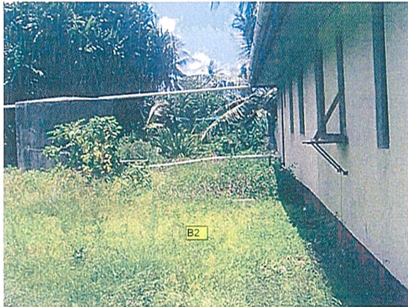
Photo(1): Area B2 (Dynamic Cone penetrometer test locations)
