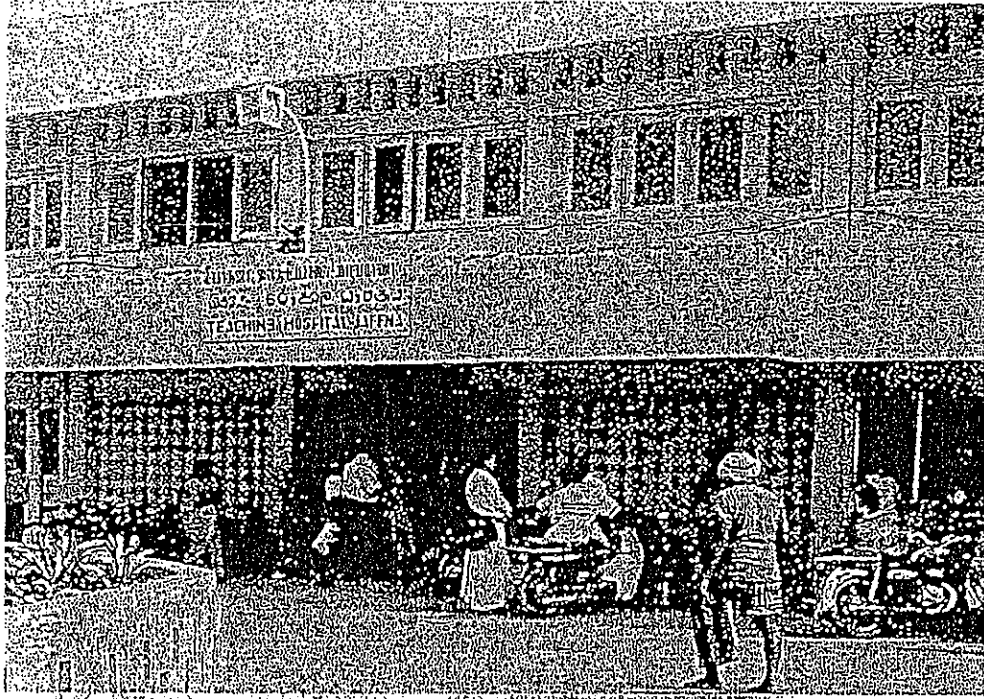
Front Elevation of Jaffna Teaching Hospital
